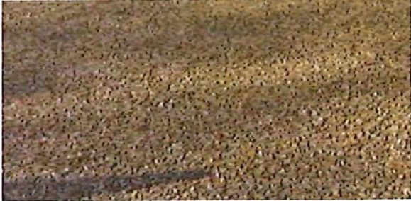
Site-wide Stabilized Gravel Option (PERVIOUS)
