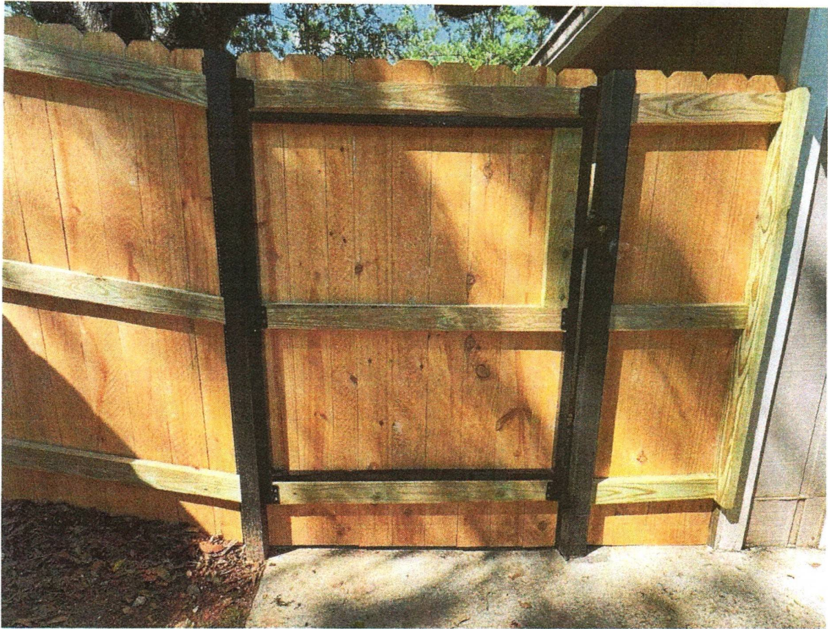
Steel gate posts and steel gate frame
