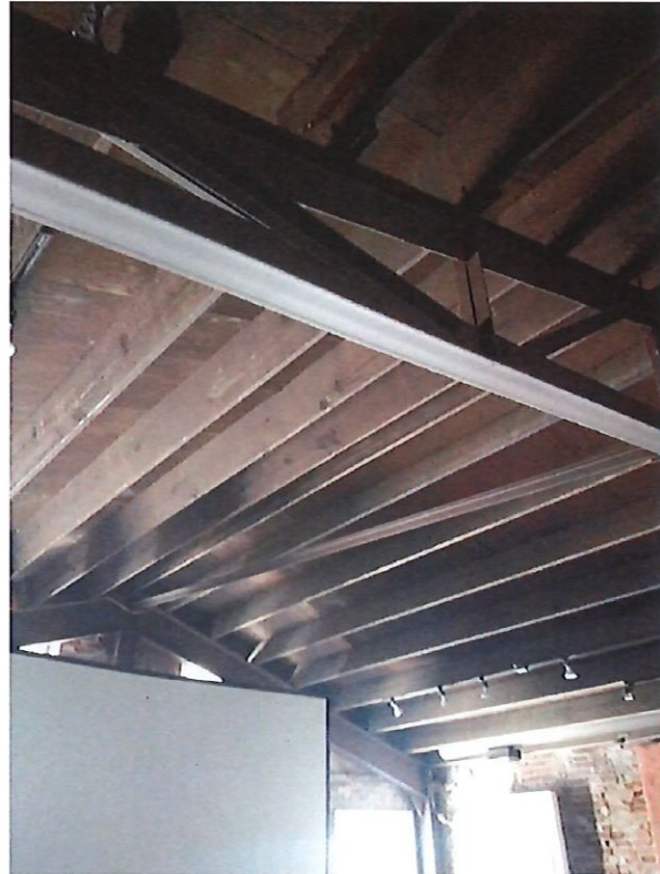
Steel trusses and lumber roof frame provide appropriate historical
