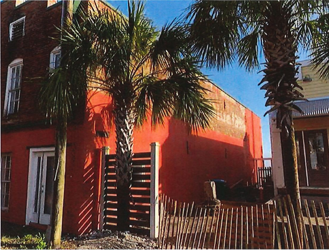
Side and rear elevation Harrison-Raney Cotton Factor & Exchange, located at 86 Water Street, Apalachicola, Florida
