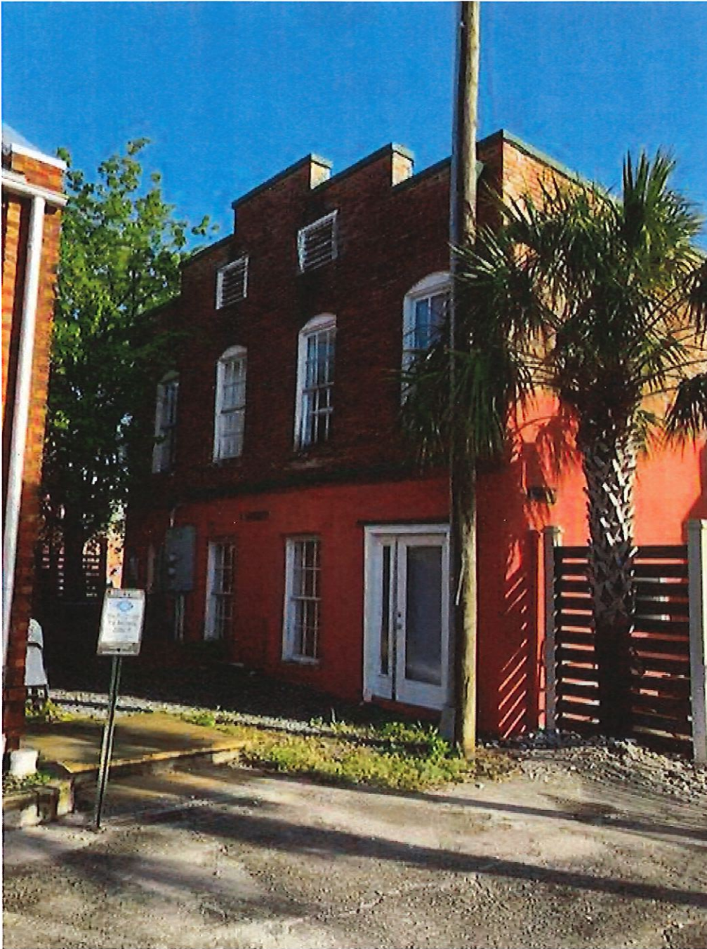
Rear Elevation Harrison-Raney Cotton Factor & Exchange Building 86 Water Street, Apalachicola, Florida
