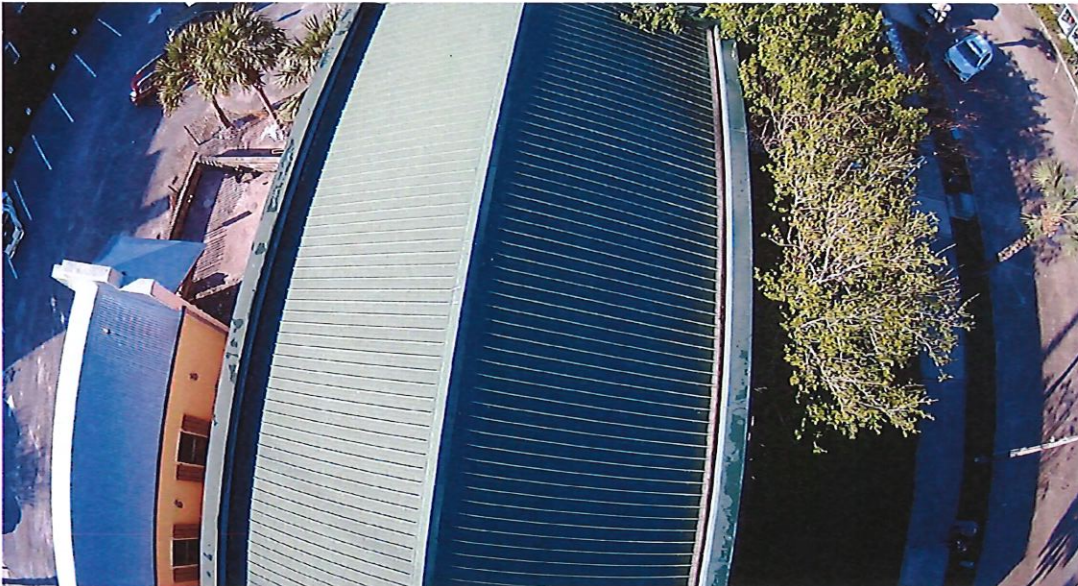
Roof surface of Harrison-Raney building, 86 Water Street Apalachicola, Florida
