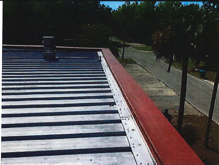
Overview of roof.
