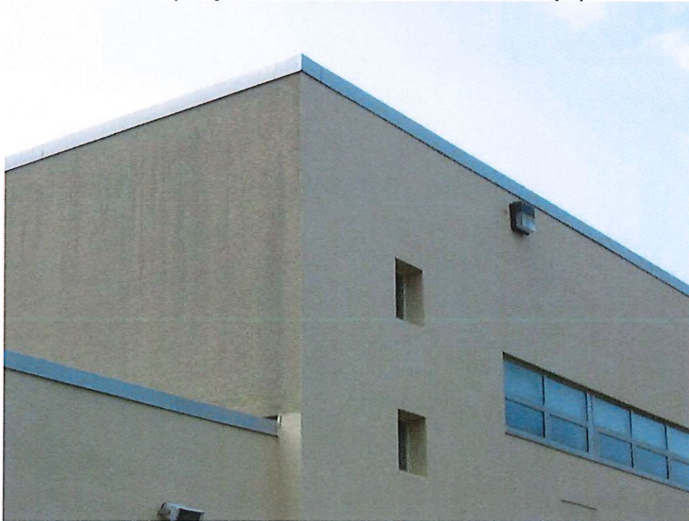
After (Only Front Wall Was Included in Scope)
