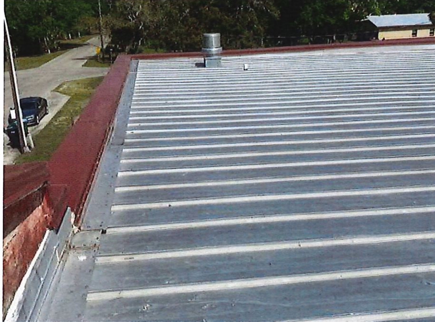
Overview of roof.
