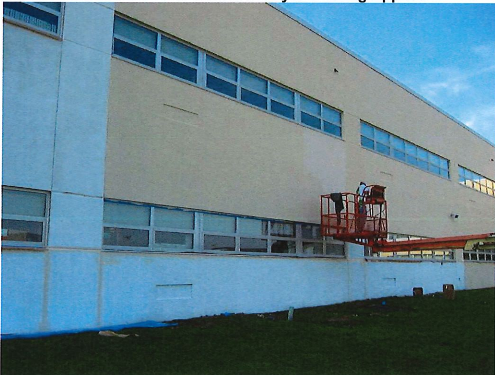
Two Coats of Breathable Acrylic Coating Applied
