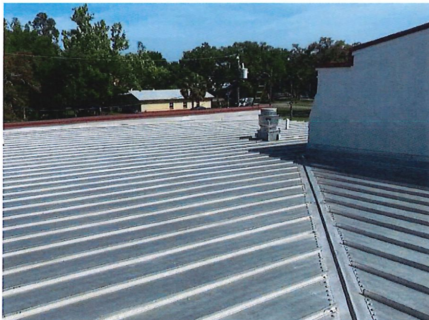
Overview of roof.
