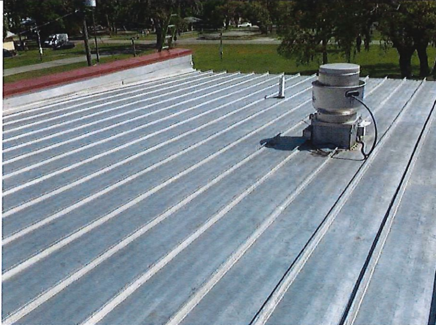
Overview of roof.
