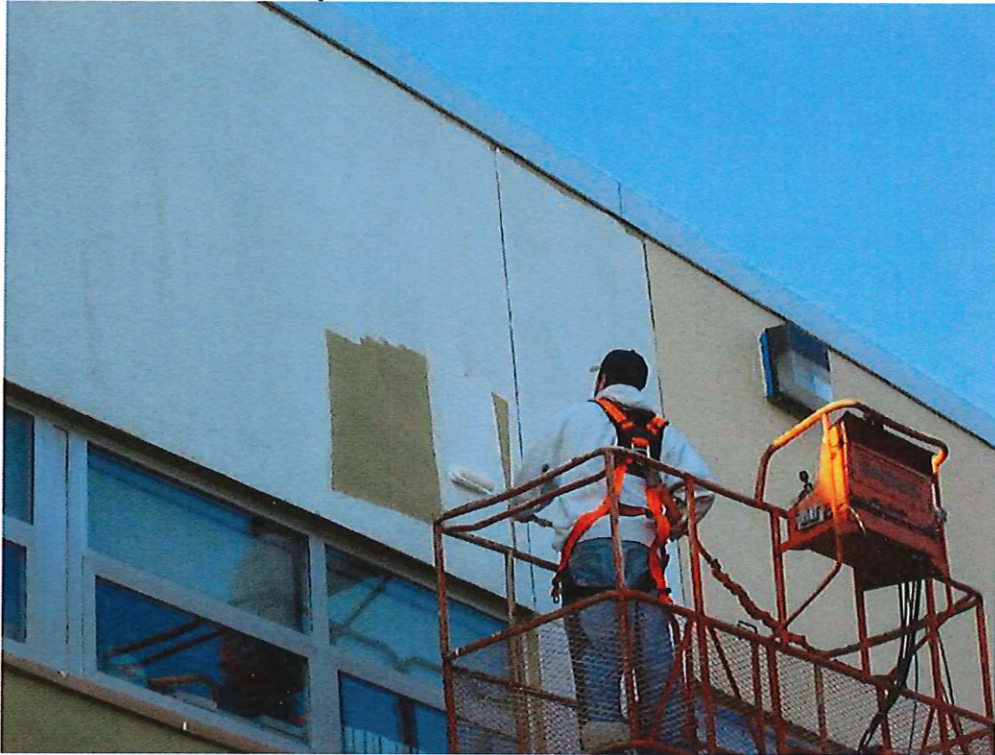
Two Coats of Breathable Acrylic Coating Applied
