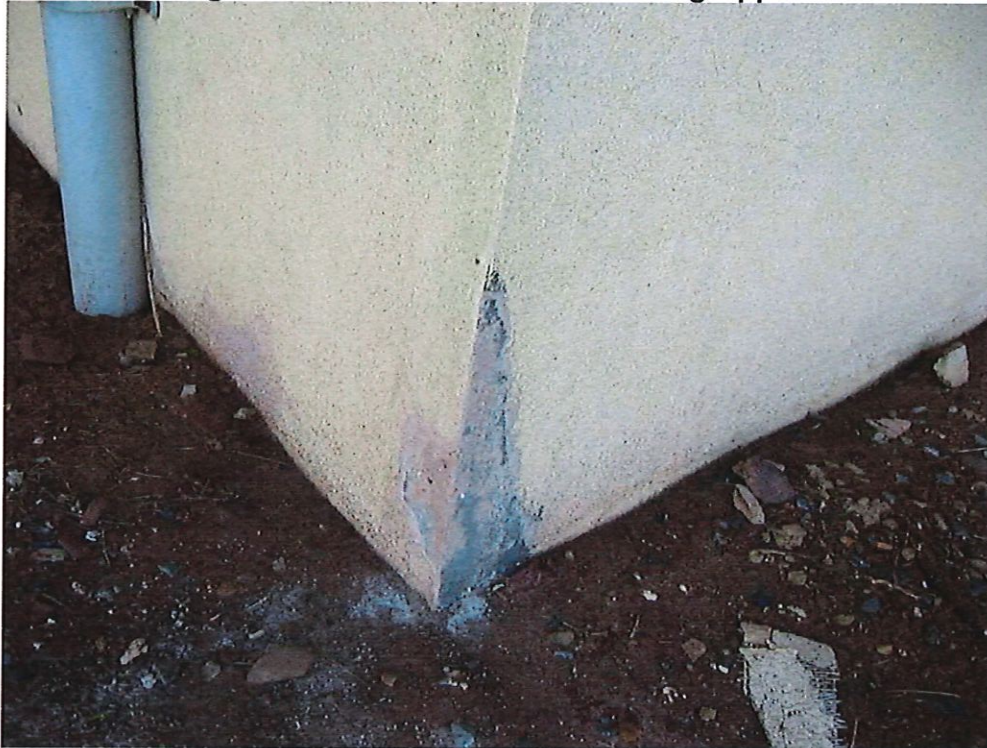
Relief Joints Caulked Prior to Coating Application
