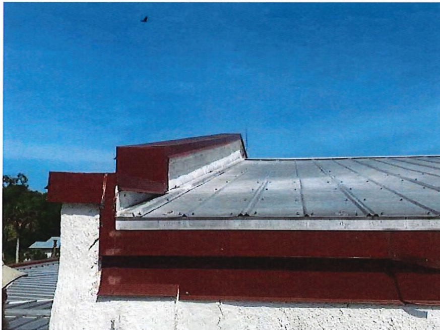
Overview of roof.
