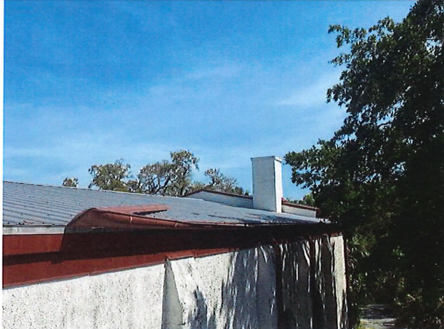
Overview of roof.
