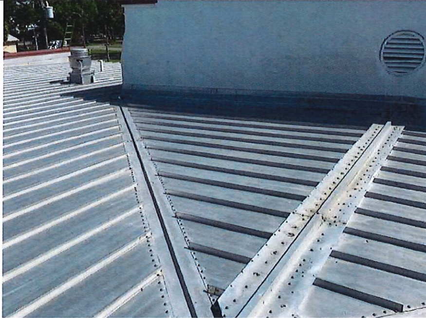
Overview of roof.
