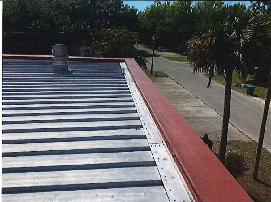
Overview of roof.
