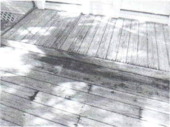
11. Both side decks - Steps over three steps high should have a handrail.
