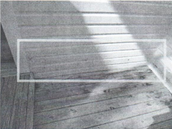
21. Wood rot noted on exterior siding: rear deck siding right of the kitchen patio door.
