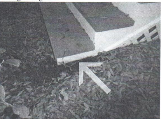
12. Master bedroom deck - Wood rot noted to the step stringers at grade.
