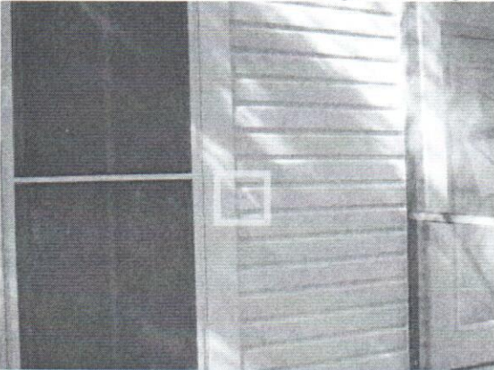
24. Wood rot noted on exterior siding: rear siding left of the screen cage.
