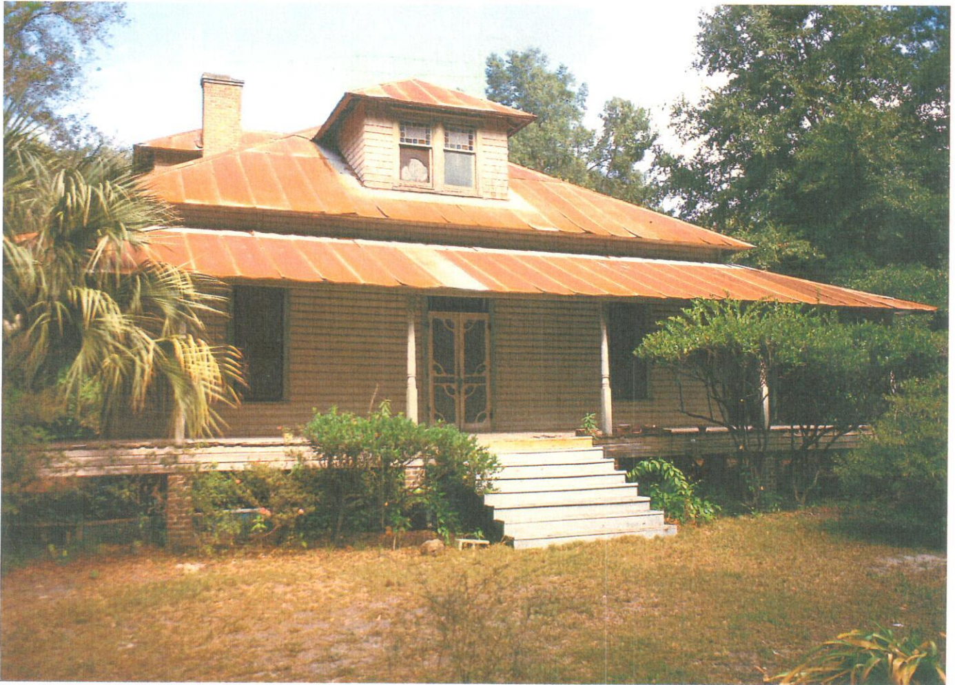
The Geiger residence in Micanopy, Alachua County, was built on the site of the old East Florida Seminary in 1908. Structural timbers from the former schoolhouse were reused for sills in this four-square Georgian residence.
