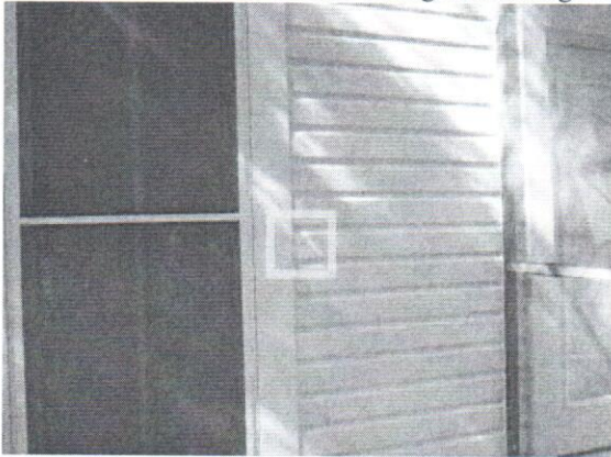
25. Wood rot noted on exterior siding: right rear corner siding below the roof to wall intersection.
