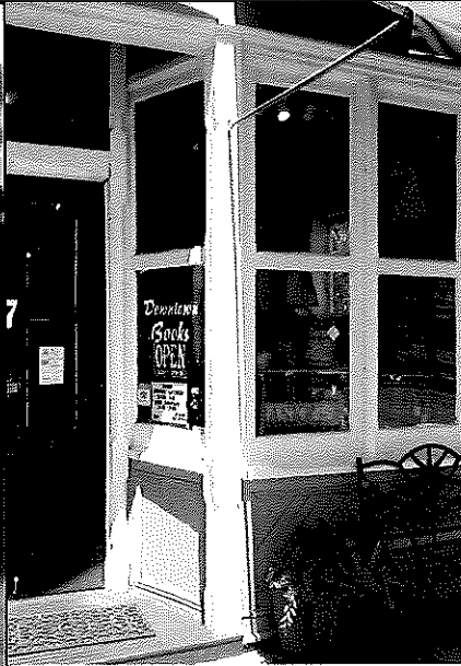
3 EXISTING FRONT ENTRANCE
