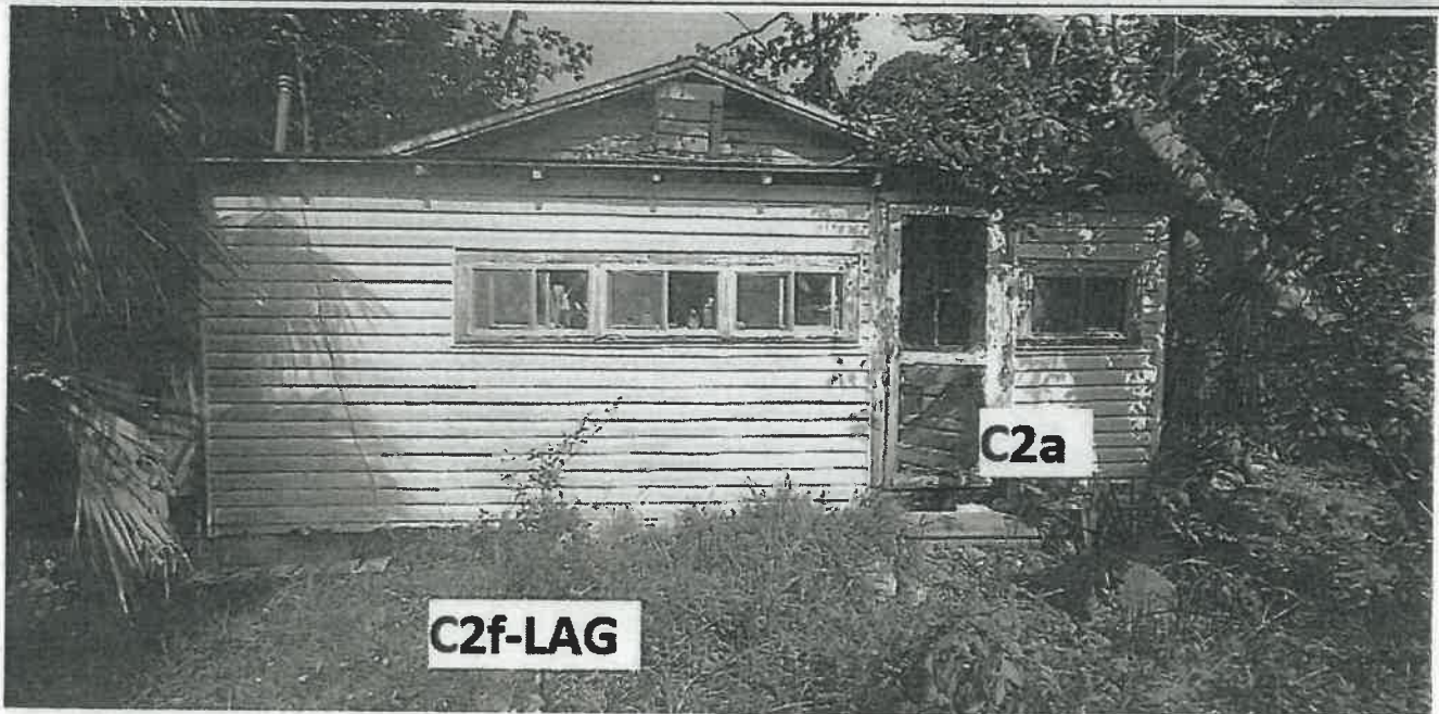
Photo Two Caption Clear Photo Two
