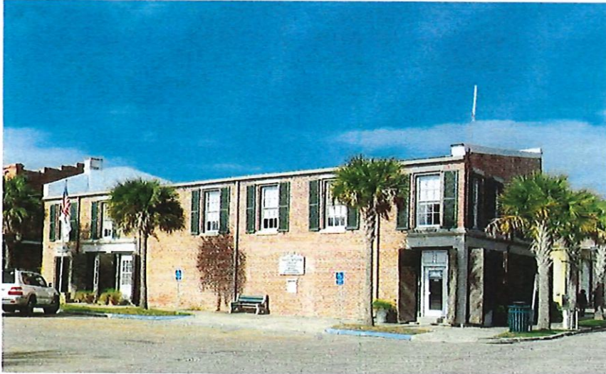
East Elevation Middlebrook Cotton Warehouse, formerly Apalachicola City Jail and City Hall
