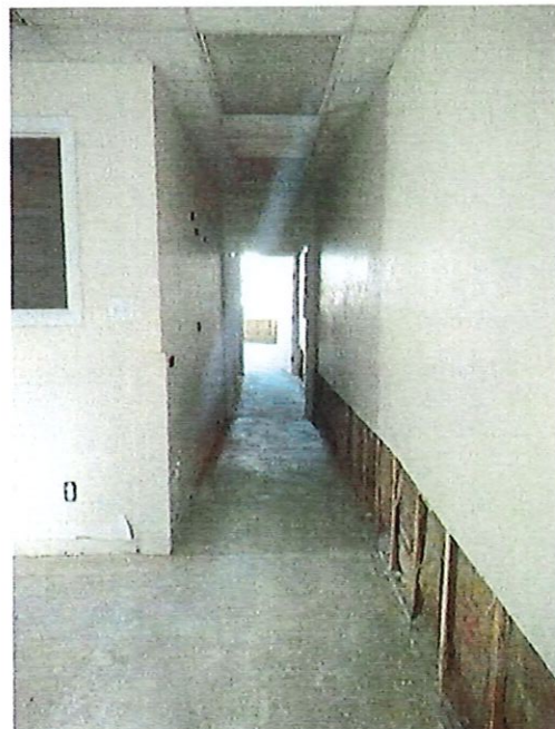
Ramp to lower floor level from central part of building. This area once served as the Apalachicola City Jail
