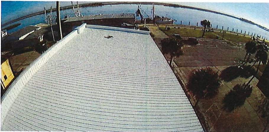
Roof surface of Middlebrook building, 1 Avenue "E", Apalachicola, Florida
