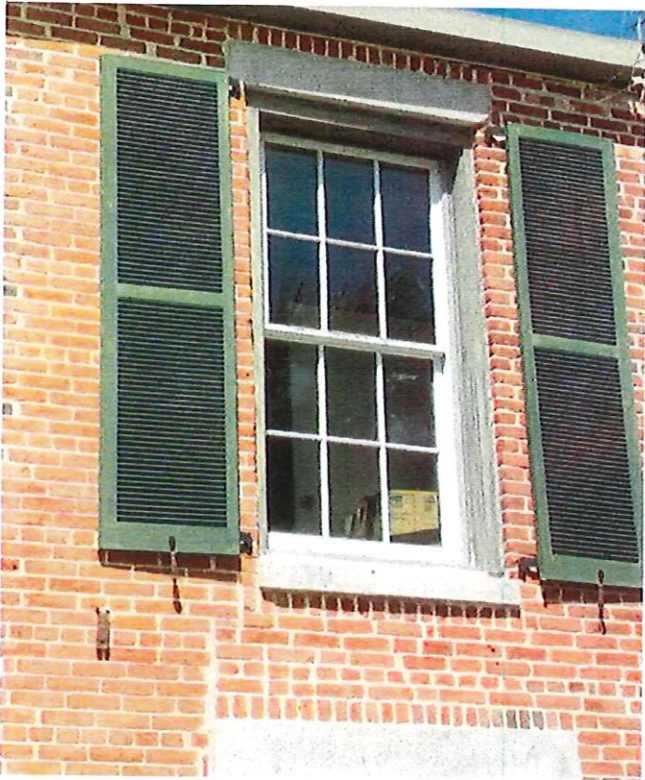
Second Floor historic windows on Middlebrook Building with operable storm shutters
