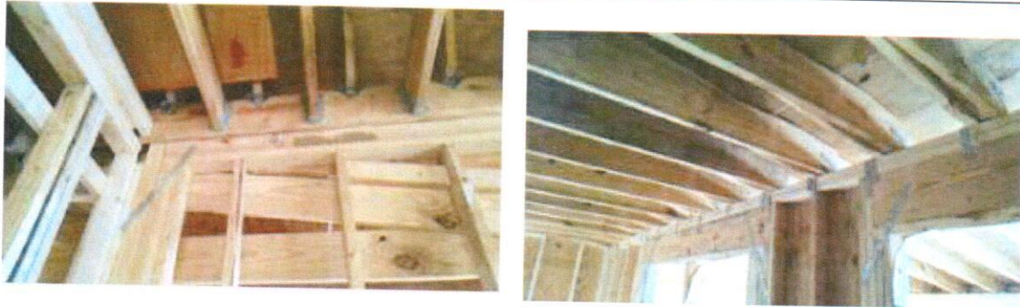
Strapping and hold downs
